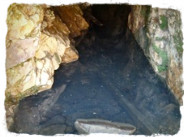
Drainage from an abandoned mine
